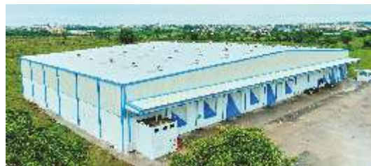
Completed PEB Structure
