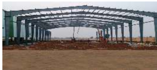
Skeleton Structure Erection
